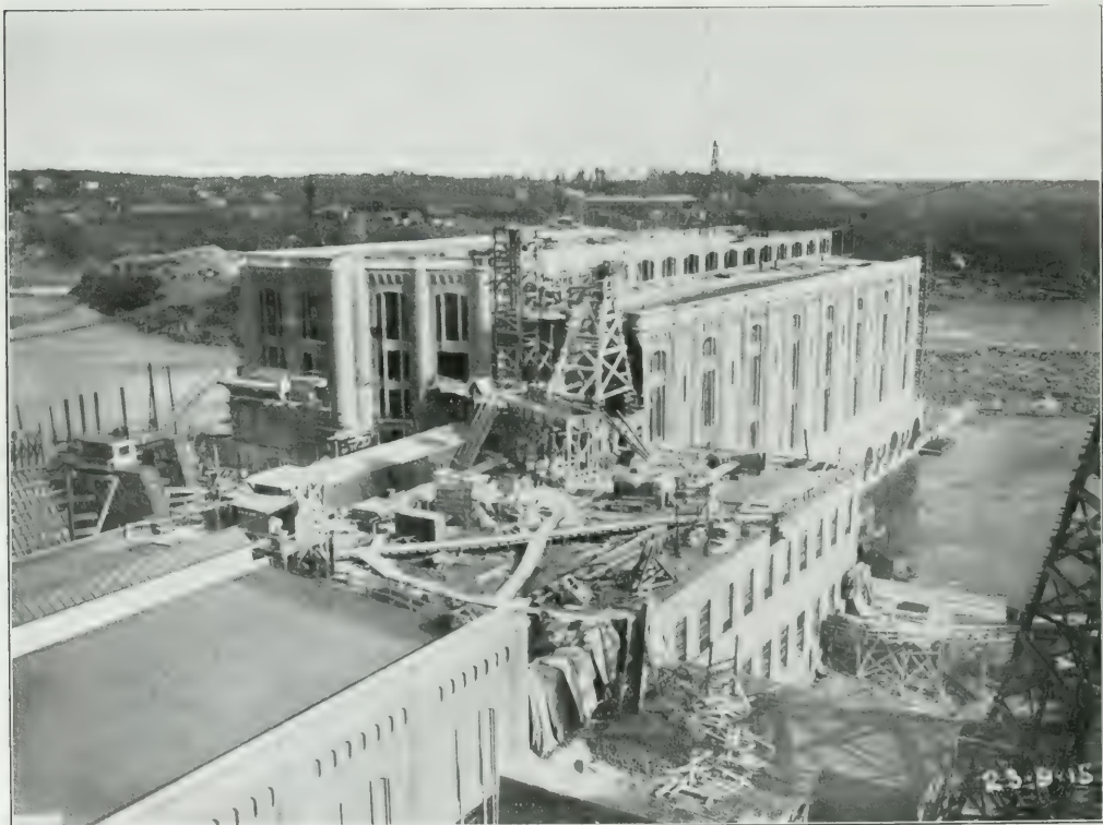
LAURENTIDE COMPANY'S LIMITED, NEW POWER PLANT AT GRAND MERE.
